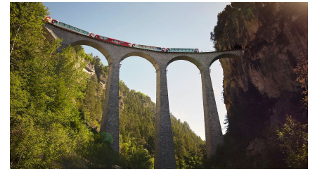
Viaducto de Landwasser. © 2023 by Glacier Express AG - Stefan Schlumpf.
